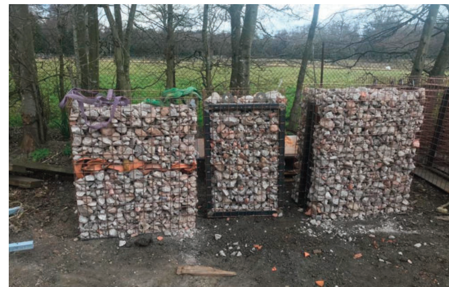
Gabions being filled with recycled aggregate. Reproduced courtesy of Richard Curle.
